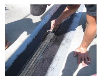
8. Repeat the process until the expansion joint is completely filled on both sides. After the expansion joint is completed, carefully remove the protective duct tape and protective paper. Do not leave this material in place during the cure, as it will not be easily removed if allowed to set overnight. Allow the material to develop full cure overnight or until header material is hard to the touch.
