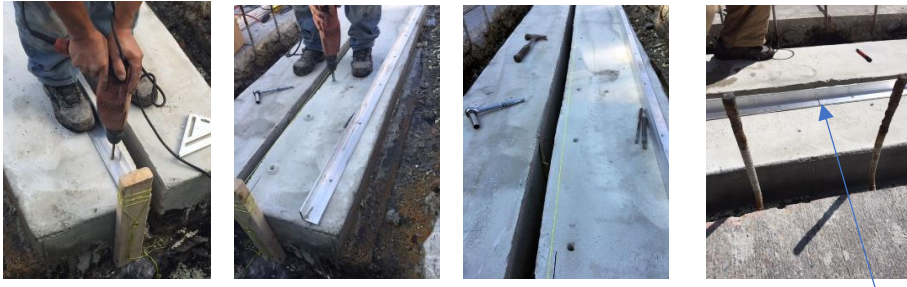
Relief cut made in aluminum angle.
