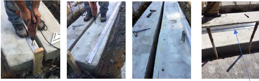
Relief cut made in aluminum angle.
