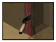
7. Silicone coating should be flush with, not protruding above, the substrate surface.
